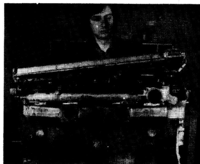
13.1. Remove camshaft covers
